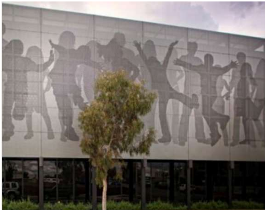
Perforated metal cladding showing silhouettes of celebrating fans will adorn the sides of the coach park
